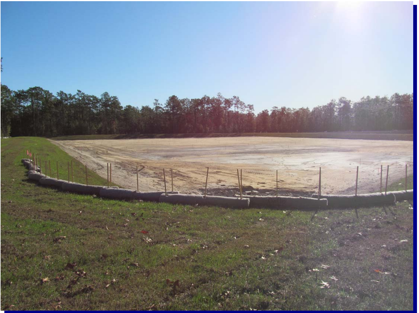
Completed Pond 2A
