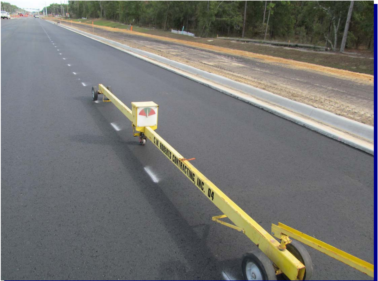
Rolling Straight Edge on Second Lift of Asphalt
