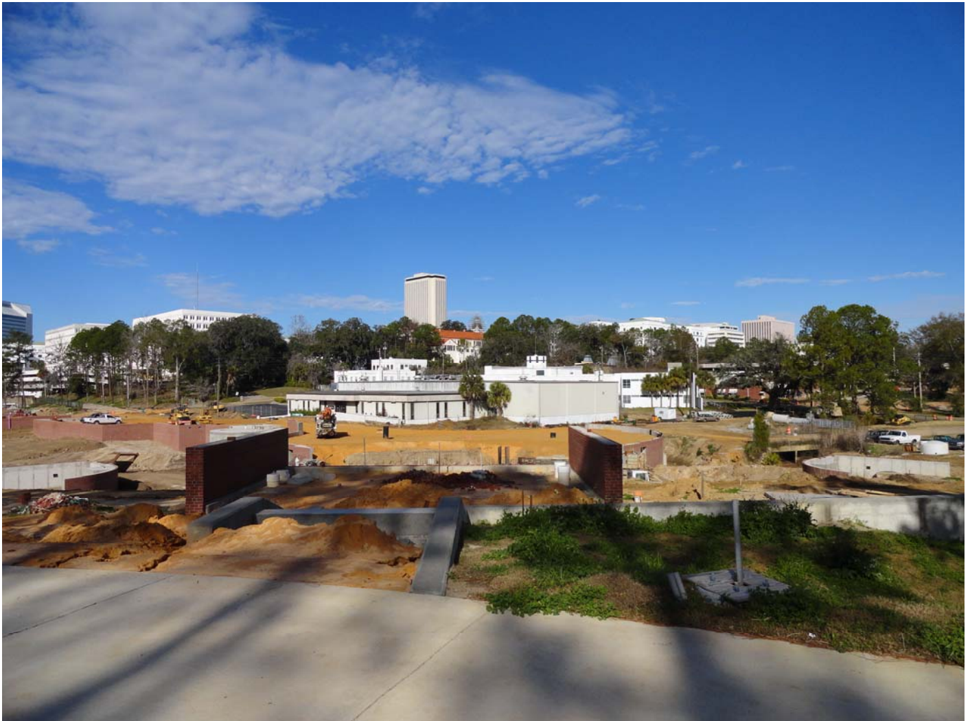
Construction of Amphitheatre
