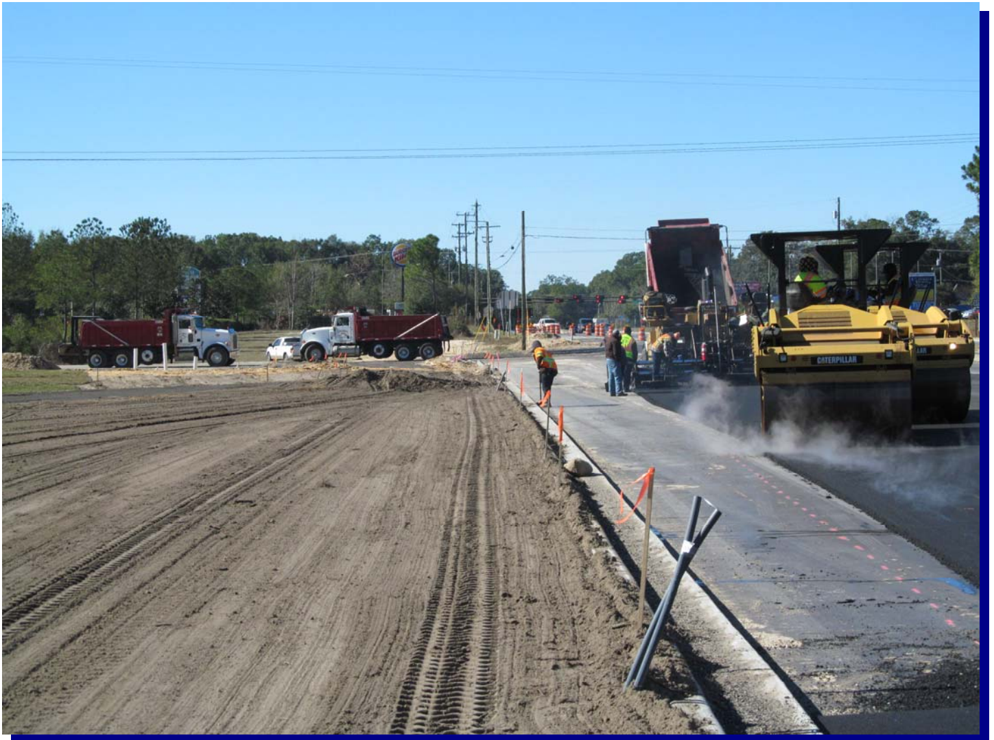
Paving Second Lift of Structural Asphalt on Eastbound Lanes
