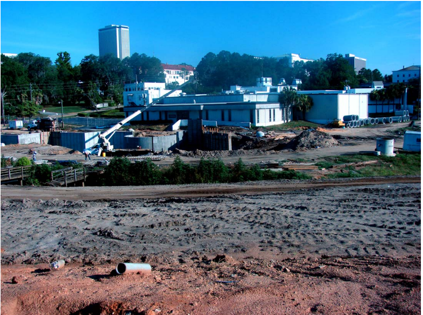
Construction of Cascades Fountain
